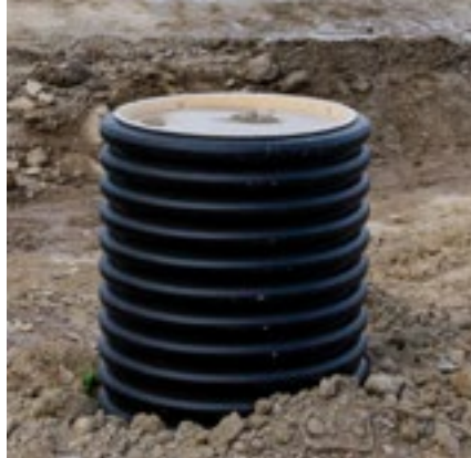
Extension pipe with temporary construction site cover
