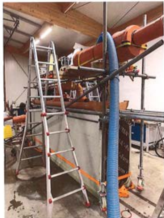
Figure 2-2: System in test set up (2)
