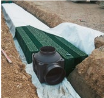
Example: target shaft with Rigofill storage/infiltration system
