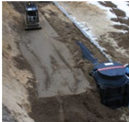
Temporary construction site cover
