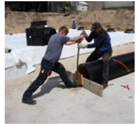
Installation of sedimentation pipe
