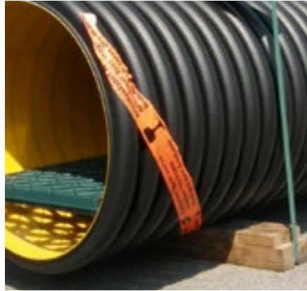
Storage on sleepers
