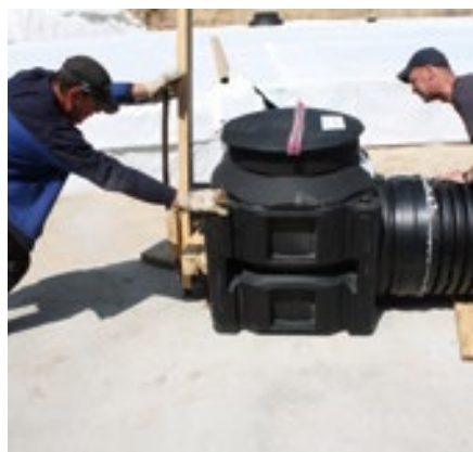
Installation of target shaft
