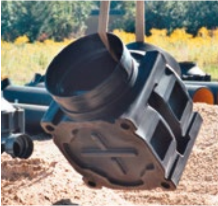
Transport using appropriate hoisting slings
