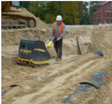
Compacting of lateral backfilling
