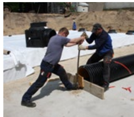
Installation of sedimentation pipe
