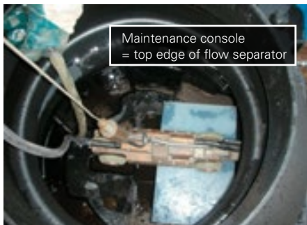
Inspection of flushing results with pan and tilt camera, camera on the maintenance console in the start shaft of a SediSubstrator L system
