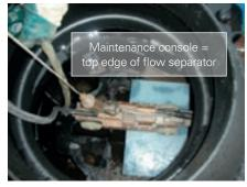
Inspection of flushing results with pan and tilt camera, camera on the maintenance console in the start segment of a SediPipe system
