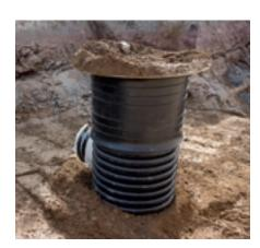
The start and target segments are delivered with temporary construction site covers.
