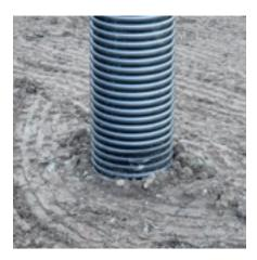
Cut the extension pipes such that they reach the support ring. Cut the pipes to length in the middle of the corrugation trough and align upright to the pipe axis using a fine-toothed saw or other appropriate tools.
