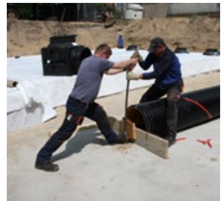
Installation of sedimentation pipe
