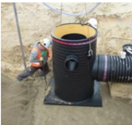
Installation of target shaft
