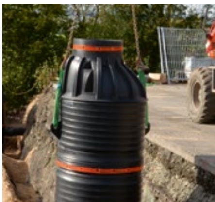
Transport using appropriate hoisting slings
