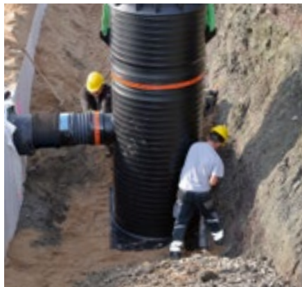
Example: target shaft with Rigofill storage/infiltration system
