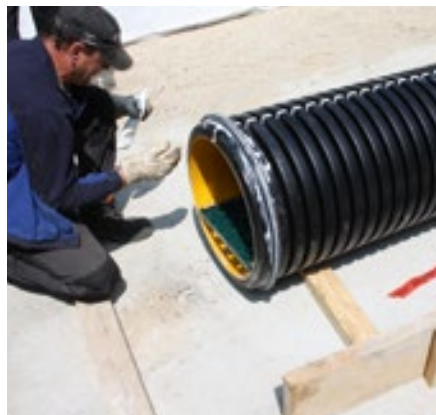
Sealing ring with lubricant
