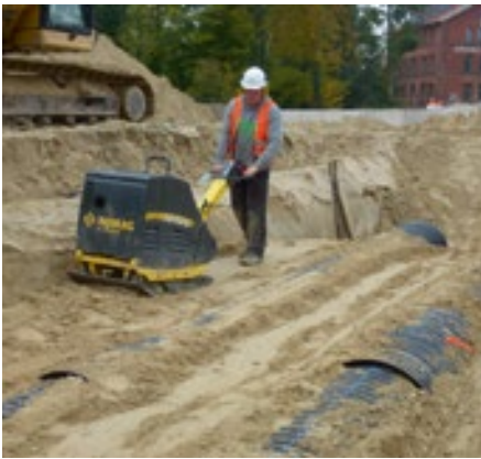
Compacting of lateral backfilling
