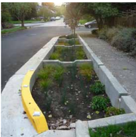
"Curb-extension" i vejside, Portland Foto: Orbicon
